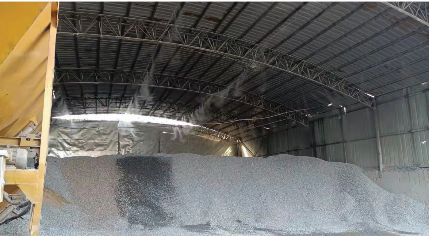
Picture 3: Spray dust reduction facilities in Hefei Factory
